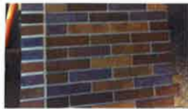
INDICATIVE IMAGE: BRICK WALL - VERTICAL STRETCHER BOND.
